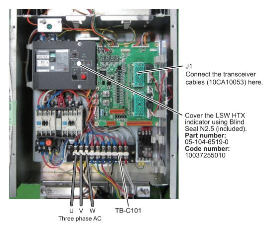
Confirm that the LED lights in red after the wiring is completed. If the LED does not light, turn off power from the mains switchboard, disconnect then reconnect the power cables, turn on the power, and check if the LED lights.
